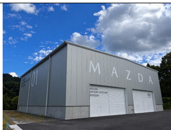
Battery Energy Storage System (MAZDA BATTERY STATION MIYOSHI)
