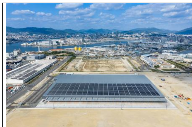
Solar Power Generation Equipment at Mazda KD Center (On-site PPA)
