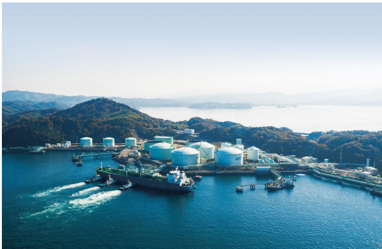
(Photo Credit: Namikata Terminal Company)
